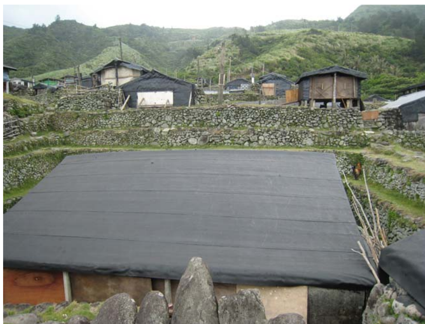
Figure 1. Traditional three-element housing unit: a semi-subterranean house (front), a work house (left), and a roofed platform (right).
